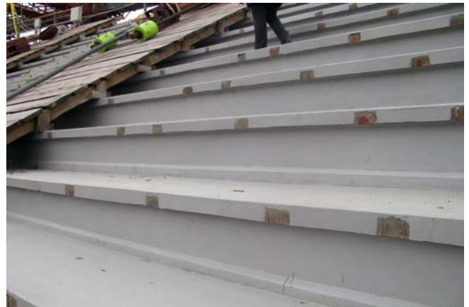
Fig. 3. Folding panel appearance after finishing repair and restoration works
