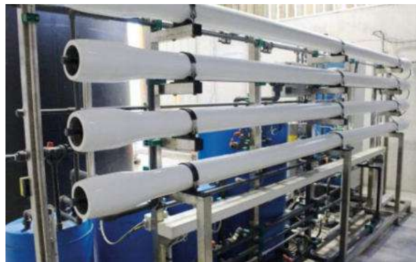
Figure 7 – Membrane filtration process with reverse osmosis modules [3]
