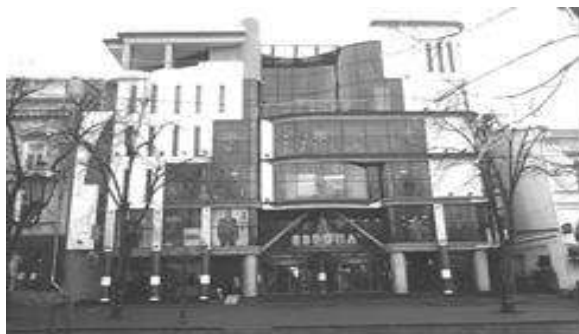
Fig. 16. Europe Shopping Center with high-tech stylistic features among the historical buildings of the XIX century on the street. Deribasovskaya, Odessa. Photo fixation of the author, 01/29/2020
