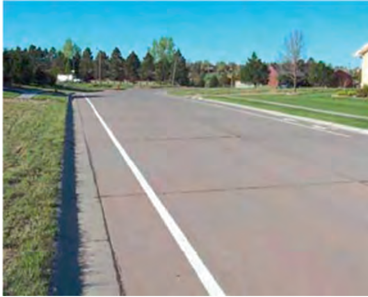
Figure 1 — RCC pavement on a local road
