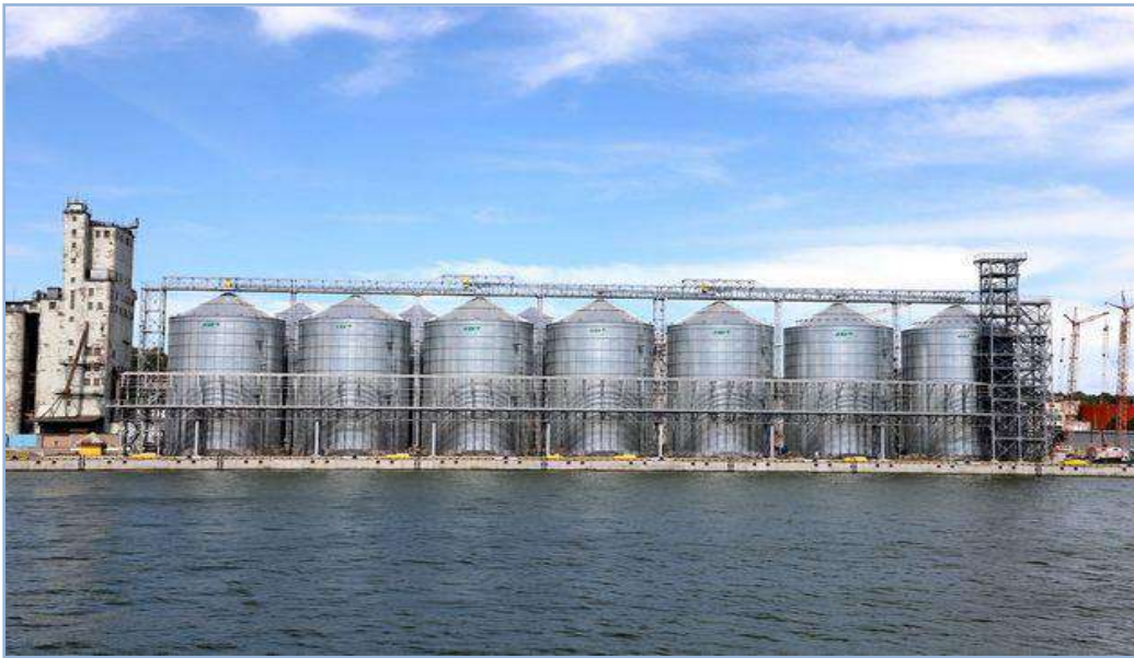
Fig. 5. Modern silos of the grain terminal of the Mariupol Sea Port [16]
