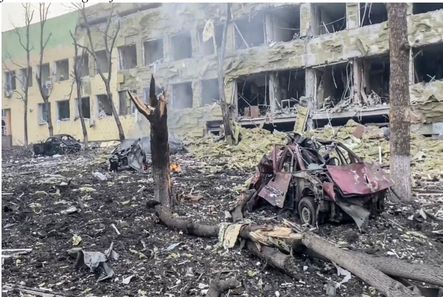
80% of residential buildings in Mariupol have been damaged. AP
